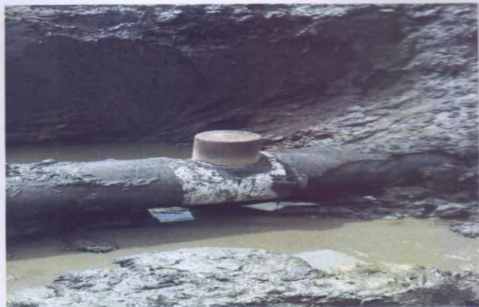
Figure 2: Wrapped cone on the pipeline.
