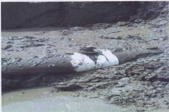
Figure 1: Replace Cone on the pipeline.
